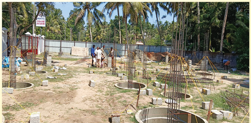
Construction progressing for Zarephath Home
